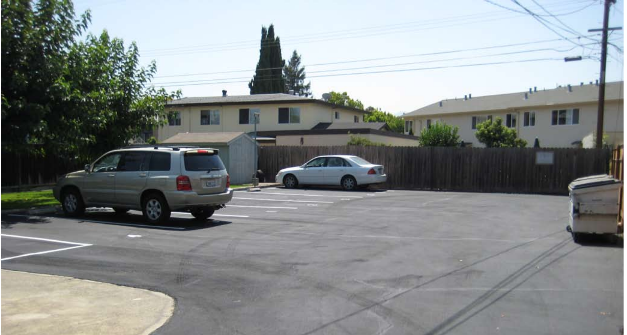
Parking lot was re sealed August 2009.
